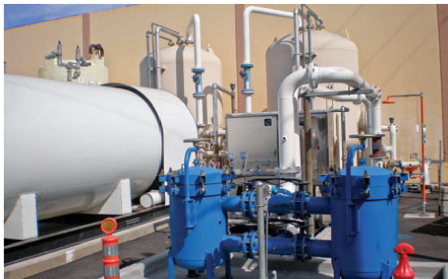
Glendale Water &amp; Power
