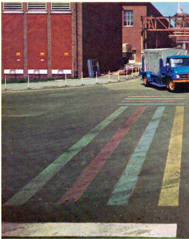
These stripes of colored road-marking asphalt were imbedded in the road surface half a year ago. Although this crossing is passed over by 500 to 600 vehicles daily, the colors have not lost a bit
