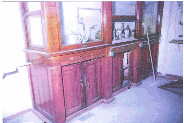
Actual Situation Fig 23: Room 335 ←N
