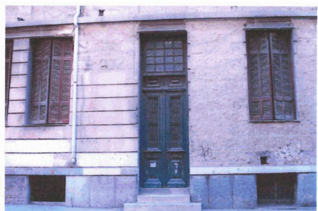
Actual Situation Fig 27: Lower Part of Western Façade
