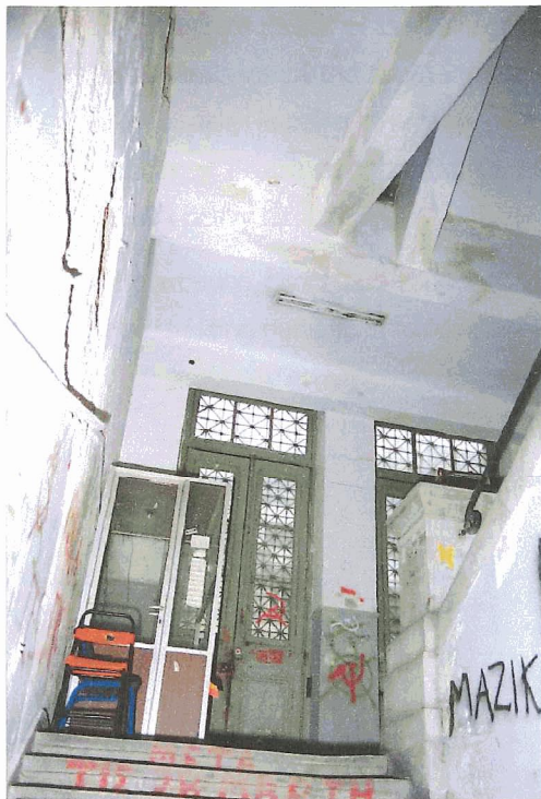
Actual Situation Fig 33: Main Staircase (From R041 to R100) ↓N
