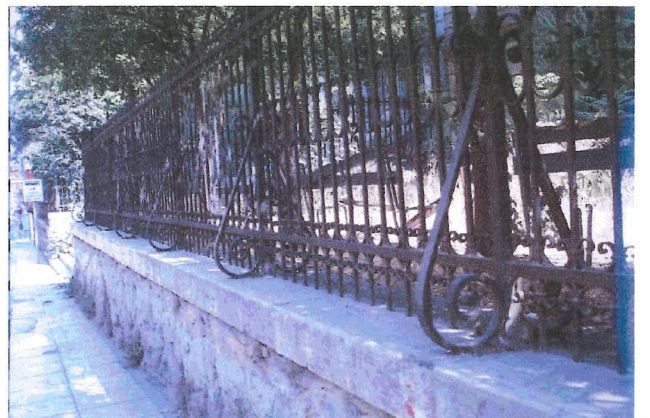
Actual Situation Fig 32: Massif Iron Railing of the Fence
