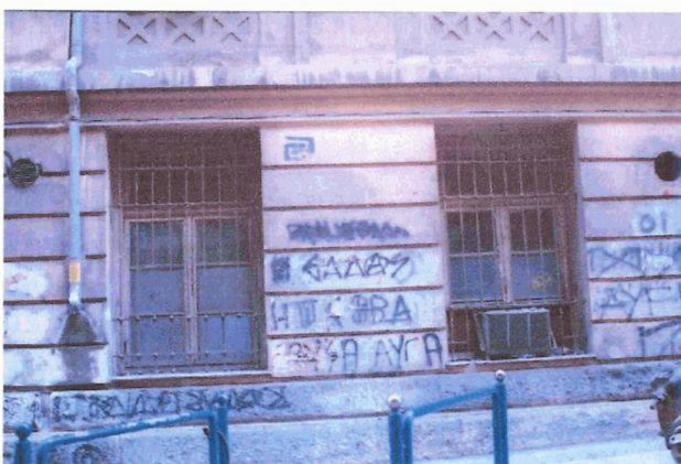
Actual Situation Fig 26: Lower Part of Eastern Façade
